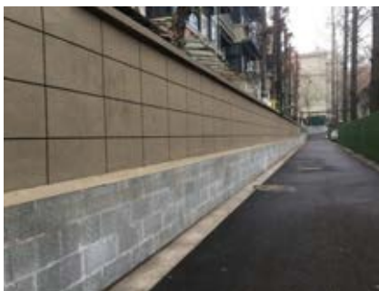
实体围墙沉闷压抑
